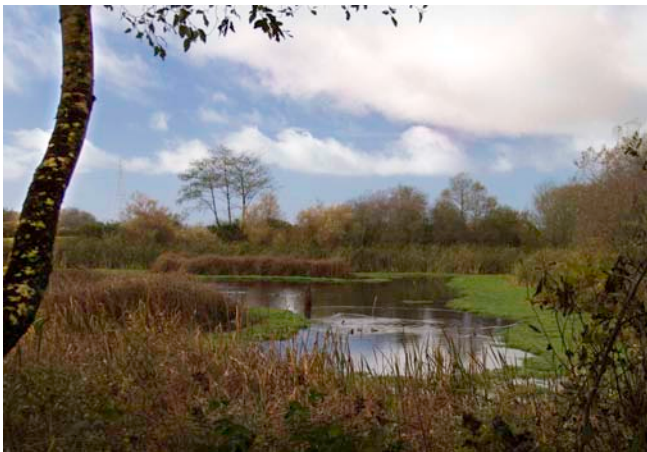
The Arcata Marsh--A wastewater treatment facility and important bird sanctuary
